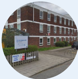
13. Medium office building, Billet Road, Waltham Forest
