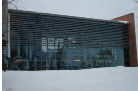
Drammen (reproduced courtesy of Star Refrigeration)
