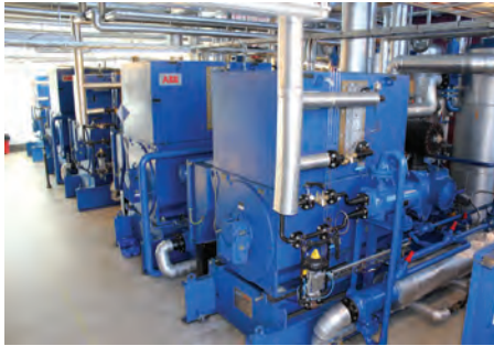
Heat pumps at Drammen, Norway (reproduced courtesy of Star Refrigeration)
