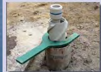
The BHE with dual pipes and a connection formed as a centralizer
