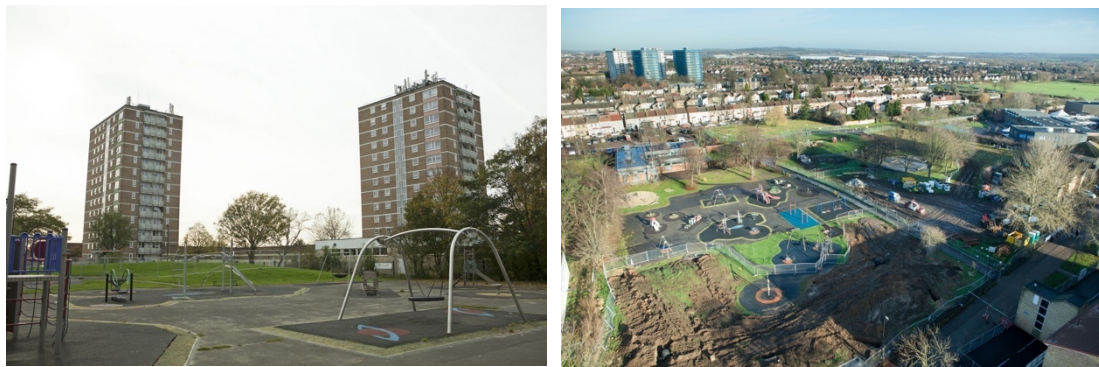
Figure 5.05 – Photographs of two of the Enfield tower blocks retrofitted with the heat pump system and of the open space where the ground array is located (© Kensa)
