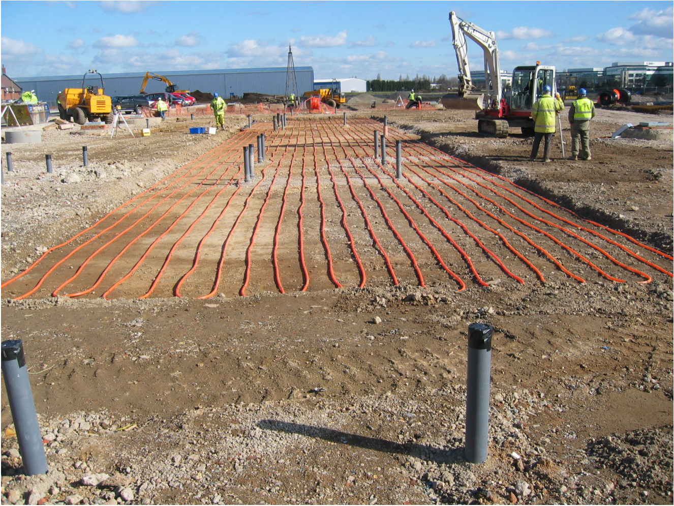
Construction of ThermalBank array (beneath the school)
