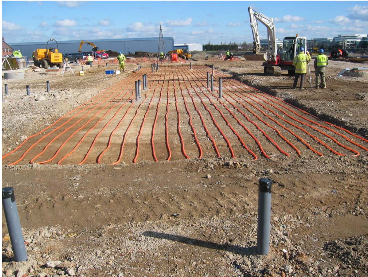
Construction of a ThermalBank array (beneath the school)
