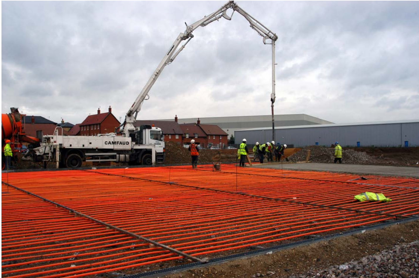
Construction of the Solar Collector array beneath the playground
